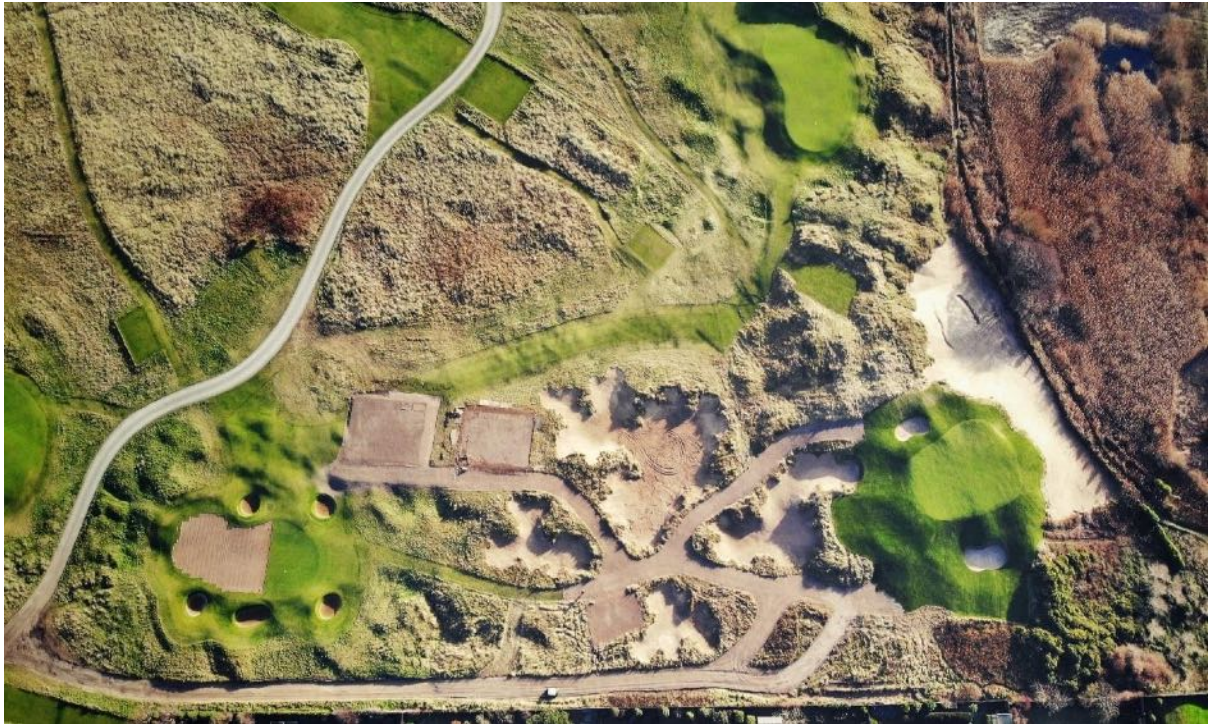
Championship 17th; Aerial View of Construction Site
